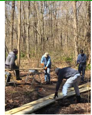
The Prvyn Sanctuary work crew constructing the puncheon walkway.
