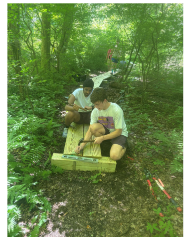
Scouts building a new puncheon walkway at Prunyn Sanctuary, Summer 2025.
